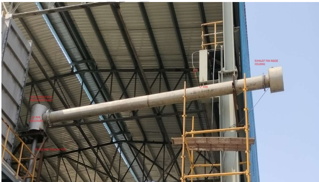
OIL MIST FUMES DIVERSION ARRANGEMENT
